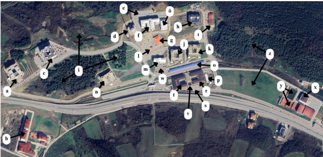
Figure 1. Yalova University Campus satellite image Buildings shown with letters in the figure letters a, n, f, h, k, j, r, o, t, classrooms and academic buildings
